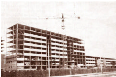
Initial construction of the New Belgrade
