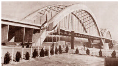
Railway-road bridge in Novi Sad
